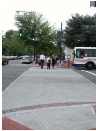
Figure 35 Stamped concrete pedestrian crossing (44)
