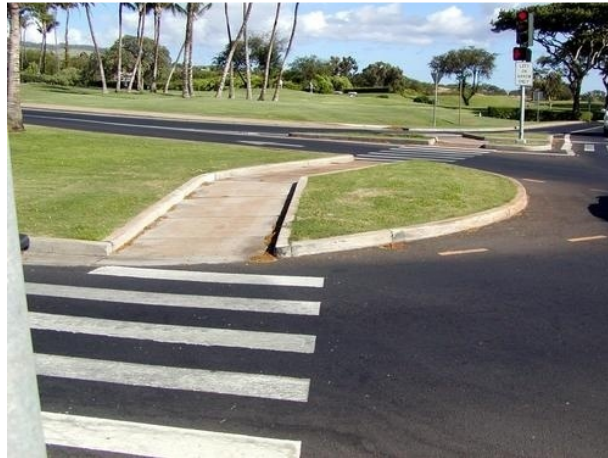
Figure 38 Pedestrian crossing island (44)
