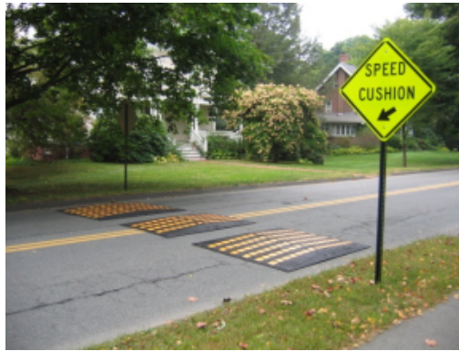
Figure 29 Temporary speed cushions
