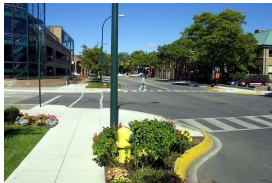
Figure 36 Curb extensions at an intersection (44)
