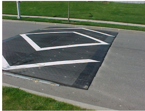
Figure 21 Temporary speed hump constructed of recycled rubber (35)
