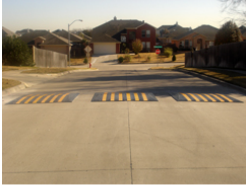
Figure 28 Permanent speed cushions (25)
